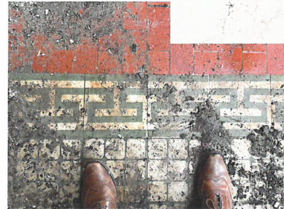
1ST FLOOR KITCHEN
