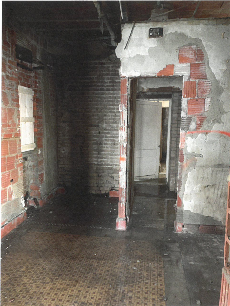
EXISTING BASEMENT DINING/KITCHEN
