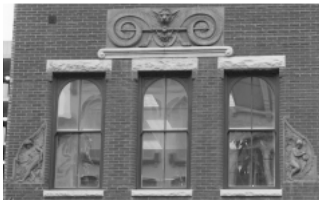
Windows are given a heightened presence through the use of ornamental stone lintels, sills, and terra cotta sculptural elements.
