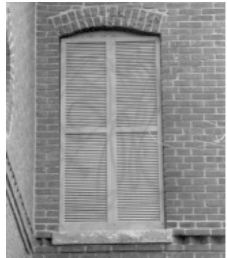
Fixed shutters are one design solution to disguise a window opening, which is no longer desired.
