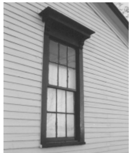
Trim helps this window to stand out from the surrounding clapboards.
