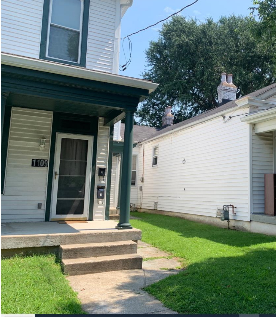
Left of subject property.
