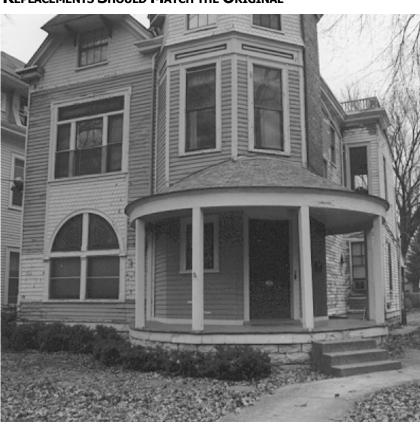
Above, the house retains it original siding, but its porch elements have been replaced by inappropriate substitutes that do not match the visual appearance of the original.
