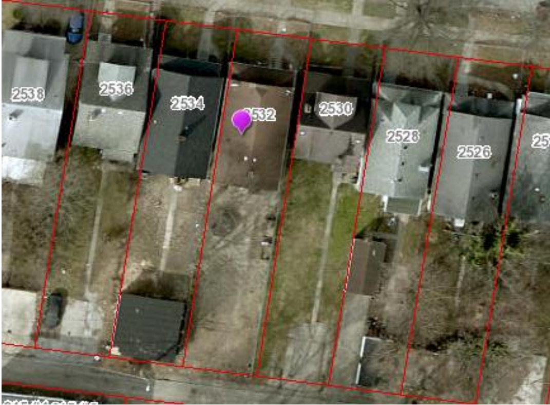
Examples of other principal structures that encroach within the required yards.
