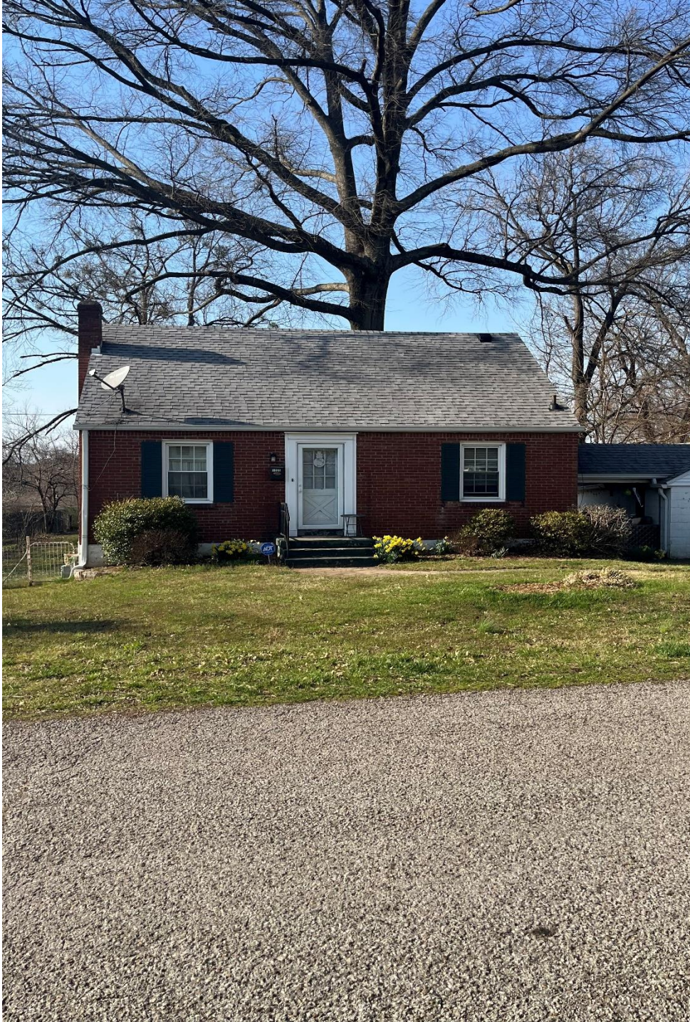
Across the street from the subject property.
