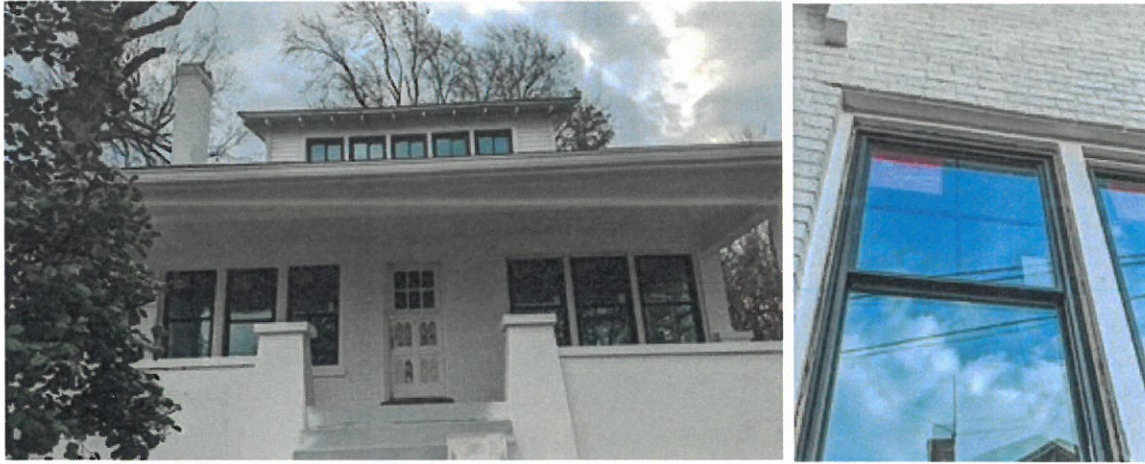
Figure 4 and 5. Replacement Windows.
