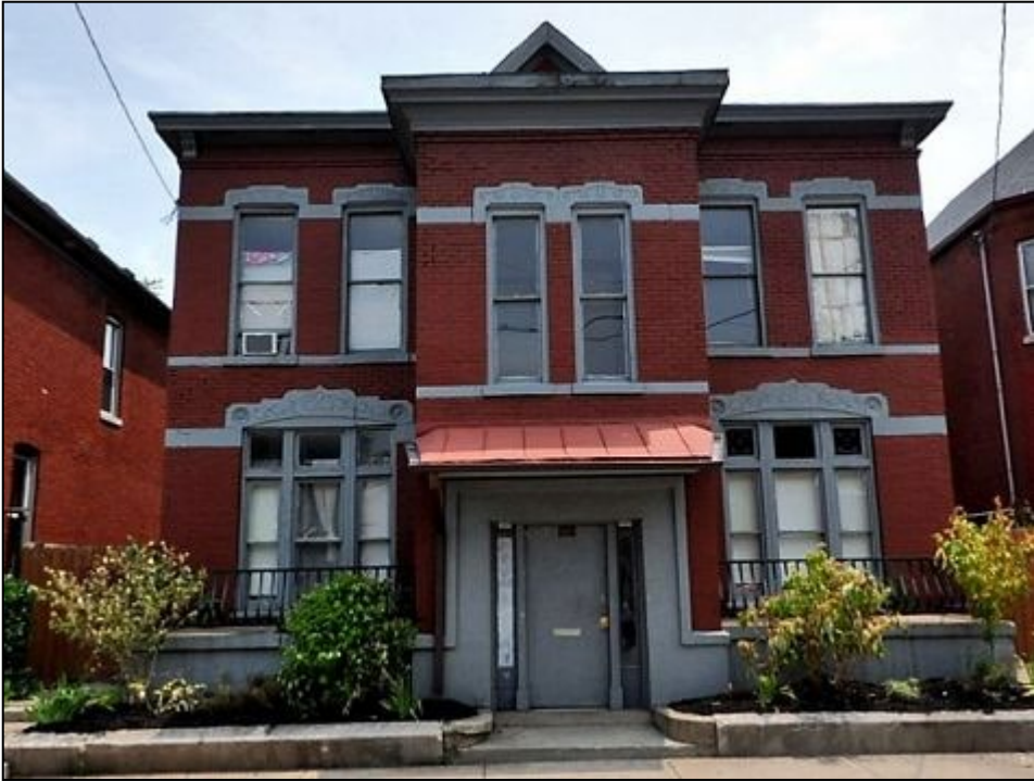
Figure 1. Photo of 1105 S. 1 st Street prior to door replacement.
