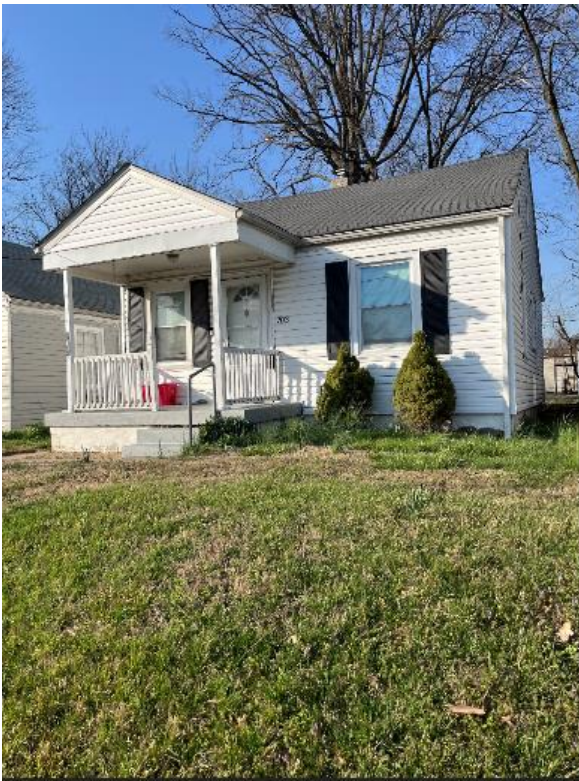
Left of subject property
