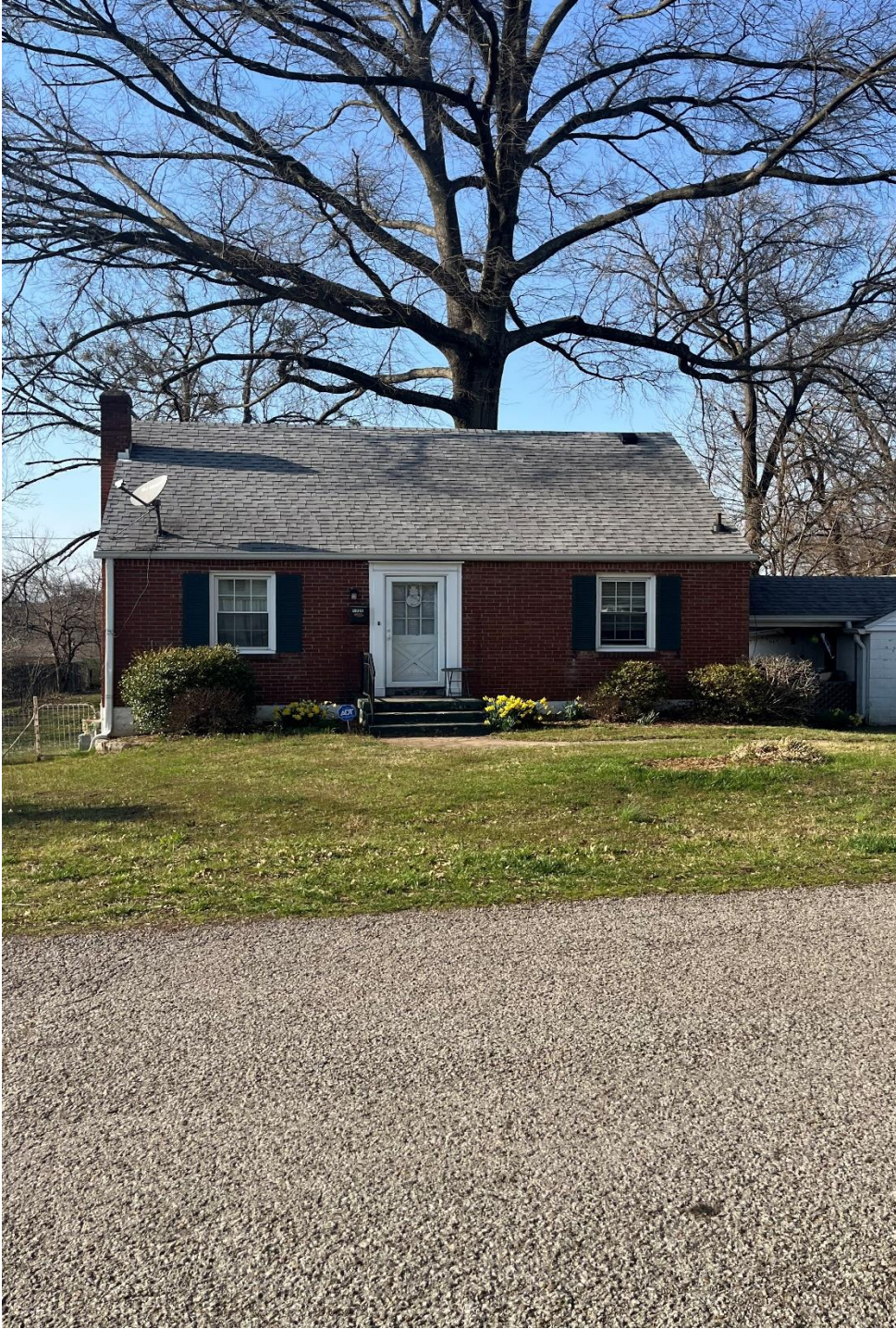
Across the street from the subject property.
